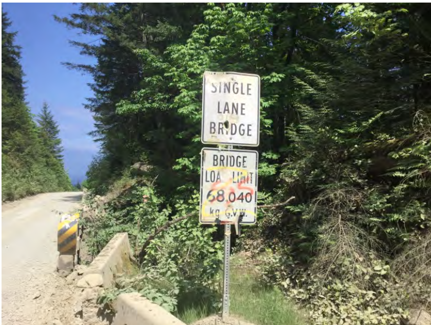
Load Rating Sign
