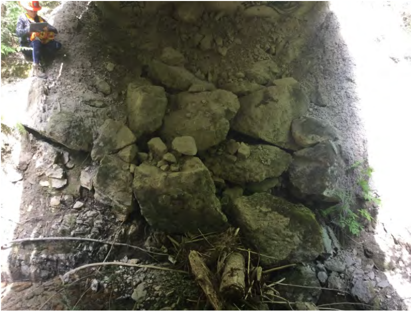
Left Bank Abutment when facing downstream
