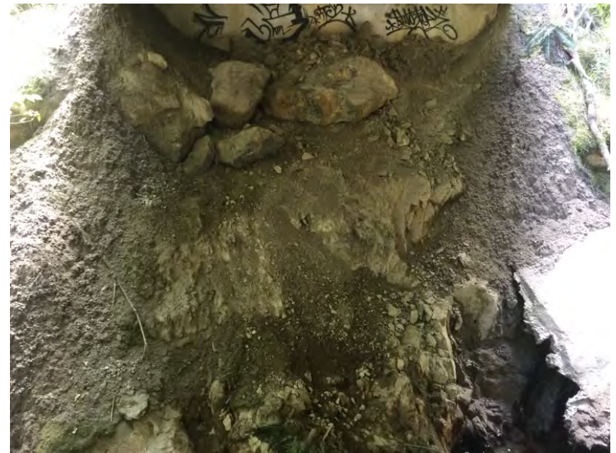
Right Bank Abutment when facing downstream
